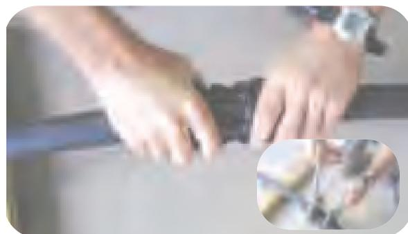
8. Hand tighten the locking collars over the threaded joint before using two pipe wrenches or multigrips (inset) to tighten the joint.
