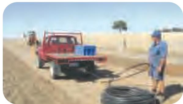
*Pipe can be unrolled along one side of the route by anchoring the outside end of the roll, tying the inside end to a vehicle with about 3-5m of rope and driving away very slowly. As pipe unrolls it should be observed for kinks. Ends should be tied down to avoid recoil.*
