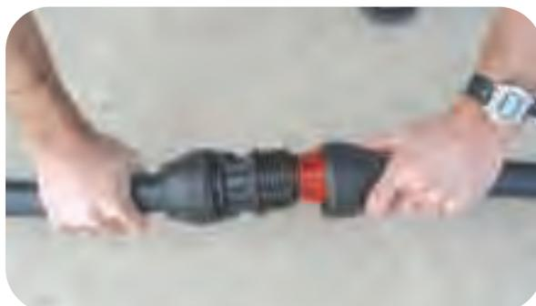
7. It is important the fitting is assembled in the correct order (above). Push both ends of the O-Ring into the threaded joint, ensuring O-ring sits firmly and is not twisted or rolled as this is crucial to the integrity of the joint.
