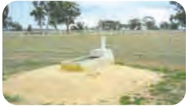
The area around each trough can be protected from erosion by placing road base material such as compacted gravel or crushed rock to a depth of 150mm. This should be maintained regularly. It is often preferable to backfill with imported gravel after stock have accessed the trough and caused a depression. Further reinforcement can be achieved by laying old car tyres around the trough and filling them with road base.
