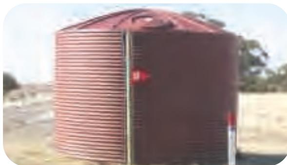
Generally, fire-fighting tanks will be 22,000L capacity, level controlled by a float valve, with hydrants consisting of twin Victorian CFA Standard couplings so that two fire appliances can be filled simultaneously.
