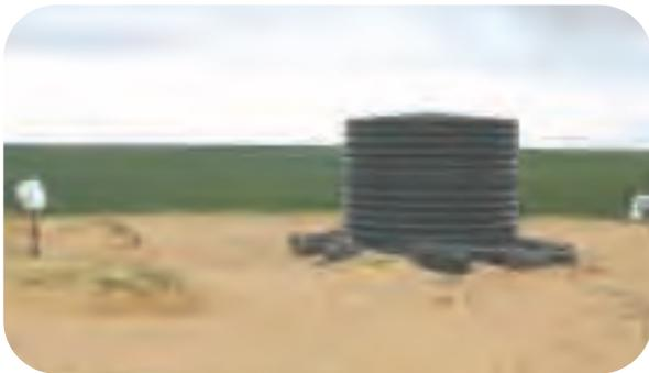
Exposed sand should be covered with 150mm of sandstone, limestone or road base to prevent wind or rain erosion. Tanks are often placed on the top of hills to make the best use of gravity. Avoid locating tanks on top of hills where soil is subject to wind erosion. Perhaps locate slightly away from the top of the rise if there is flexibility with elevation requirements.
