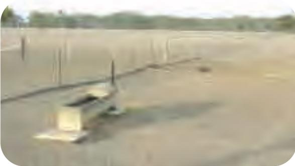
Polyethylene pipes should not be laid above ground because of the effects of temperature and physical damage.
