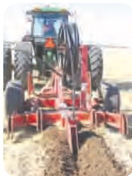
There are some disadvantages with laying pipes using rippers. It is not possible to observe the pipe in its final resting place, making it difficult to know if the pipe has been stretched as it was installed, especially when using powerful equipment. Installing the pipe at depths below 300mm can take a lot of additional work such as pre-ripping and the use of a heavy-duty ripper driven by a powerful tractor.
