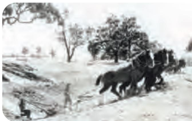
Men and horses worked side by side to build the early channels and dams. Over time, this gravity-fed system expanded to include 12 storages that divert water from the Wimmera and Glenelg rivers and various lakes. More than 17,500km of open earthen channels deliver water from these storages to over 20,000 dams.
