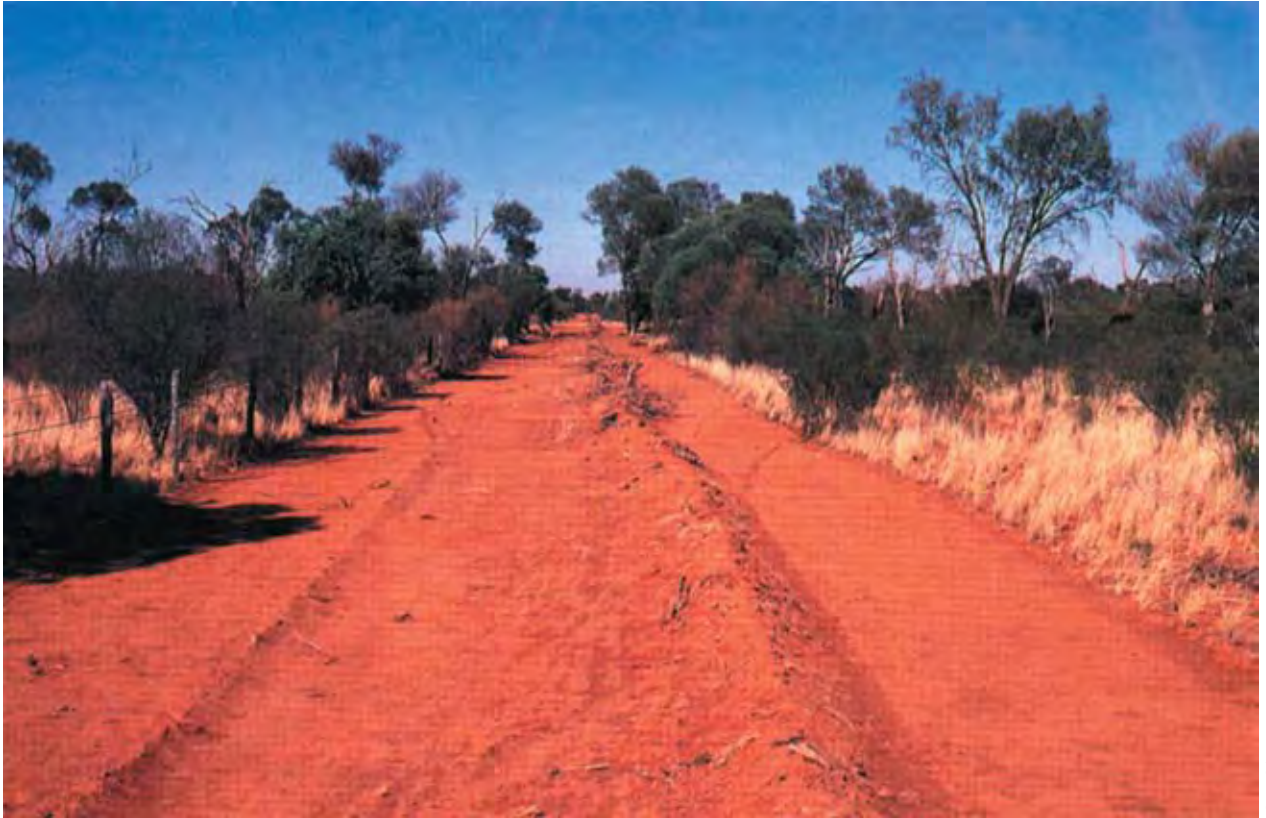
Figure 3. A well-constructed firebreak, three grader blades wide. The trash windrow was turned into the break on the last pass of the grader to leave a clean edge to burn off when lighting the burn.
